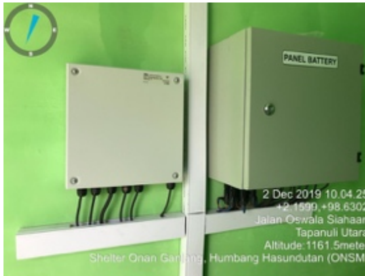
Figure 4. Panel Battery at mini region shelter
