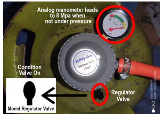
Figure 13: Second Regulator with Valve Condition After Locking
