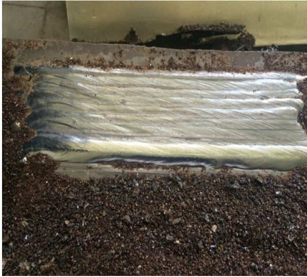
Figure 9 : Second layer of weld surface
