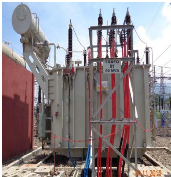
Figure 2. A 60 MVA power transformer in Bumiayu substation, Indonesia
