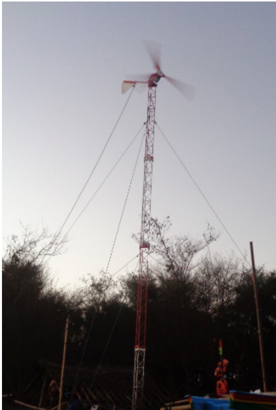
Figure 3. A 2 kW wind turbine with permanent magnet synchronous generator
