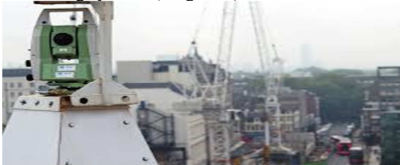
Figure 1 - Monitoring Of The Building With The Robotic Tacheometer Use
