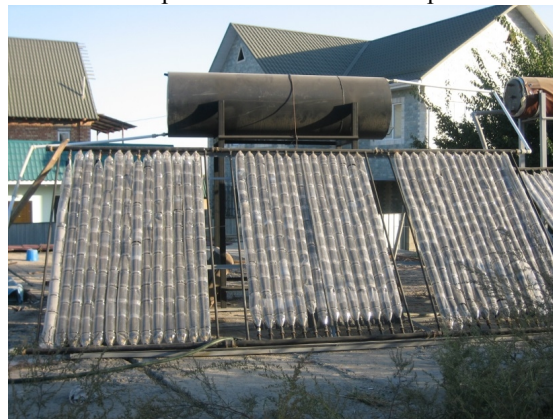
Figure 1: Getting started with GU-500 with tubular solar collectors with an absorbing screens
