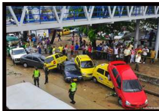
Figure 1: Piled Up Vehicles As Toys After A Flash Flood In 43th Street. May 14, 2011
