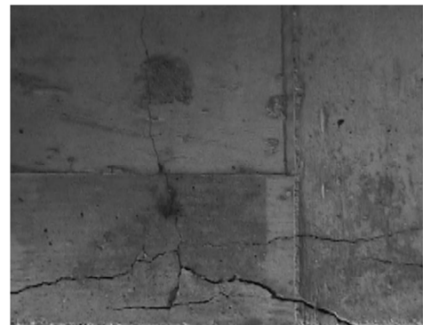
Figure. 12. Concrete Bridge Image With Alligator Crack
