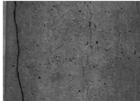
Figure.10. Concrete Bridge Image With Longitudinal Crack
