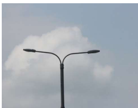
Figure 1: Different tilting of the luminaire on Cikampek and Cipularang toll road
