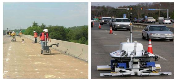
Figure 2. Testing site for bridge assessment at the Haymarket, VA, USA. (Right) RABIT - Robotic Evaluation Bridge Inspection Tool By The Federal
