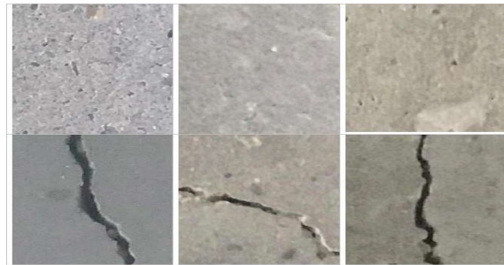
Figure 9. Concrete Crack Images for Classification. Upper row: Images with no cracks, Lower row: cracks (Source [39,40])
